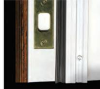
Magnetic Weatherstripping utilizes refrigerator technology to provide a durable, tight seal to provide year round comfort and energy efficiency.
