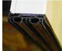
The door bottom weather-strip slides off and on for easy replacement and forms a weather-tight seal to the threshold. The result is a superior seal that keeps the inside in and the outside out.
