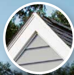
J-Channel with Aluminum Rake
