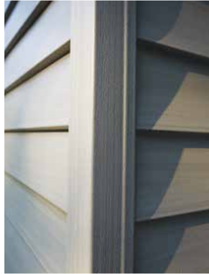
Simple Traditional Cornerpost with matching siding color for less definition.
